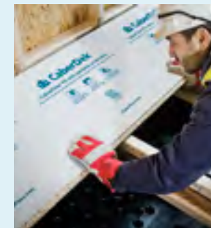
10mm minimum expansion gap should be applied to the perimeter
